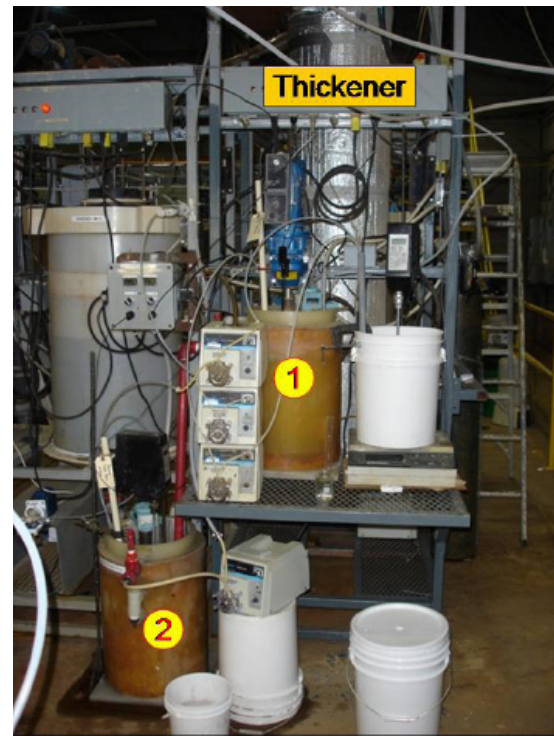
Figure 8: The 2 - Stage Iron Removal Circuit with the Iron Residue Thickener in the Background
