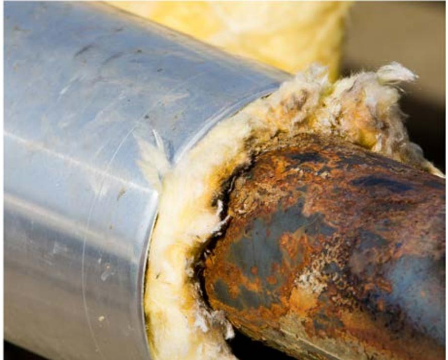
energy is “leaking” out of the system, the inspector will be more concerned with ensuring containment. Keeping heat and cold in, and keeping moisture out. The consequences for this course of action are:
